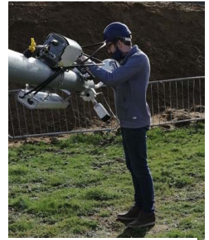
Installing prototype secure communications
